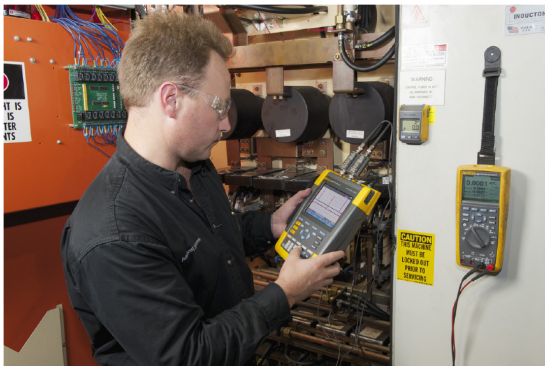
With only low-voltage control power on and the main system power locked out, Leigh uses his Fluke 190-204 ScopeMeter® and 289 multimeter to check some of the internal circuits and verify gate pulses on the large silicon-controlled rectifiers (SCRs) that switch the high frequency current.
