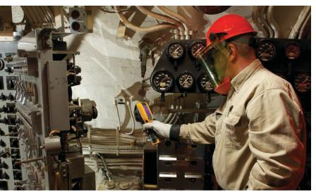
The control room is the center of the submarine, both physically and operationally. Bill uses a Fluke Ti125 to look behind the IC switchboard, which has both 120 volt ac and 120 volt dc systems.
